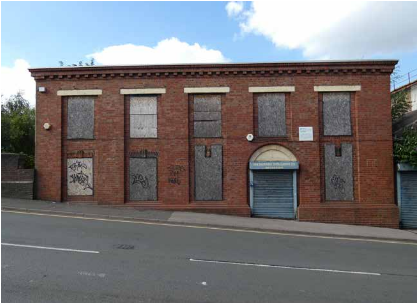
Commercial building frontages to Bridge Street
