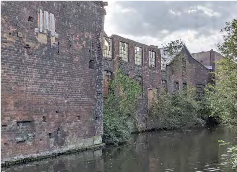
Warehouse frontages to the Engine Arm
