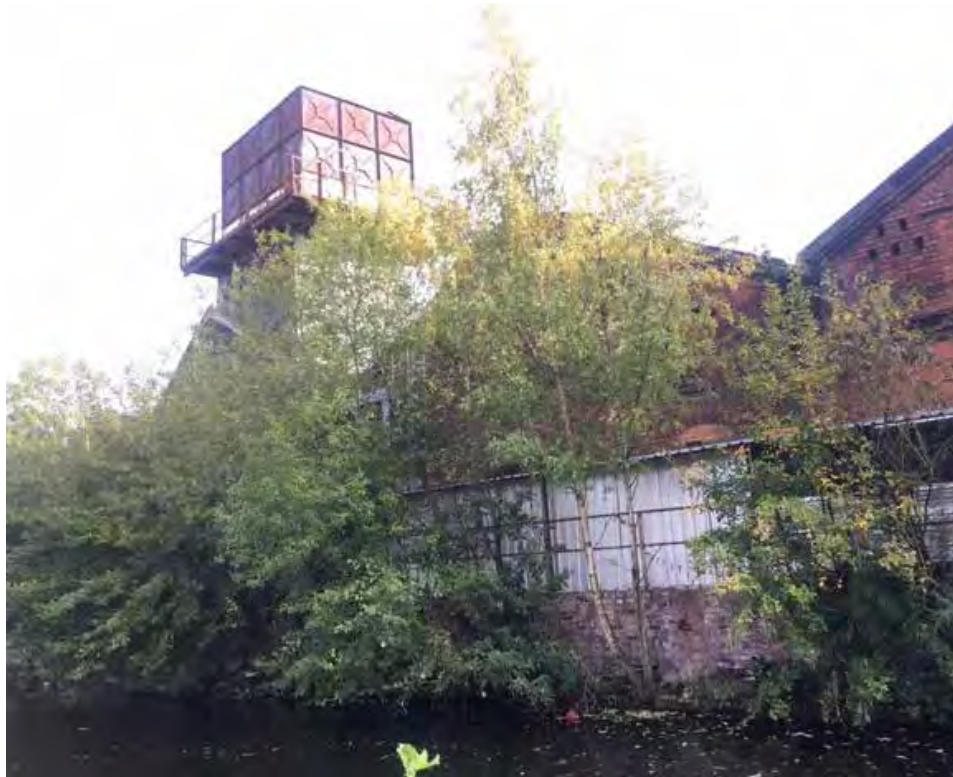
Existing water tower
