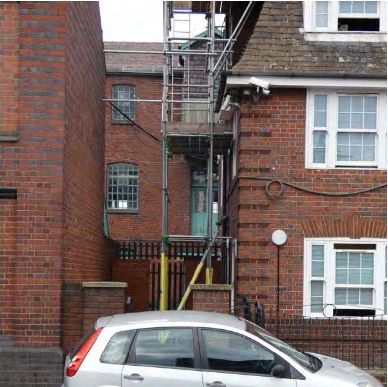
Glimpsed view of Block 300 from Rolfe Street
