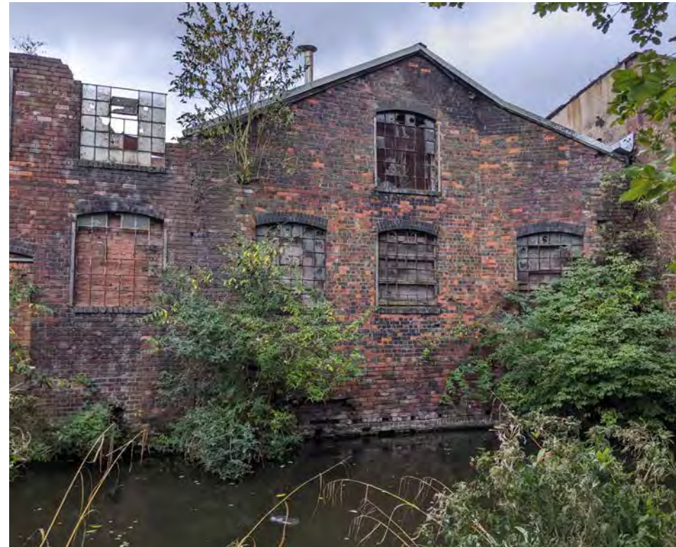
Existing warehouse elevations onto the Engine Arm
