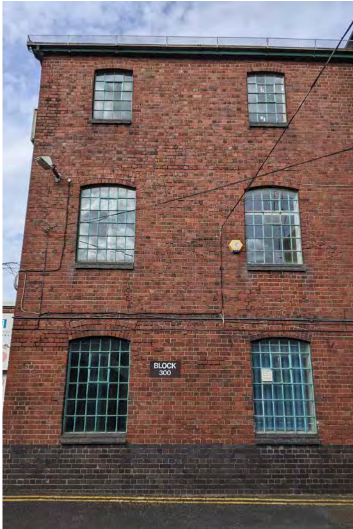
Rolfe Street – materiality and detailing
