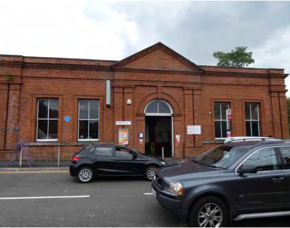
Rolfe Street station building
