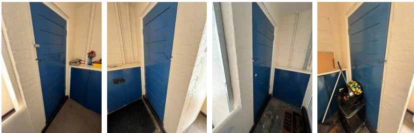
Samples of 2 nd floor storage cupboards adjacent to flats
