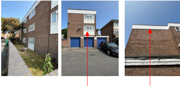
UPVC and Spandrel panelling, UPVC cladding
