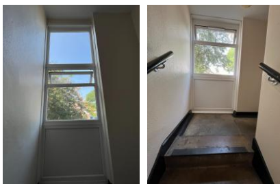
1 st and 2 nd floor landing
