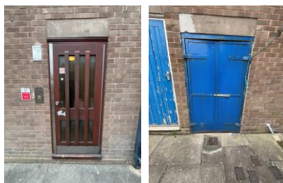
Front Entrance and bin refuse room.
