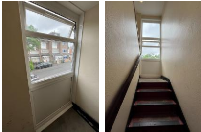
1st and 2 nd floor landing
