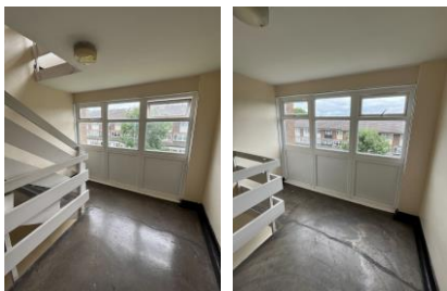
1 st and 2 nd floor landing
