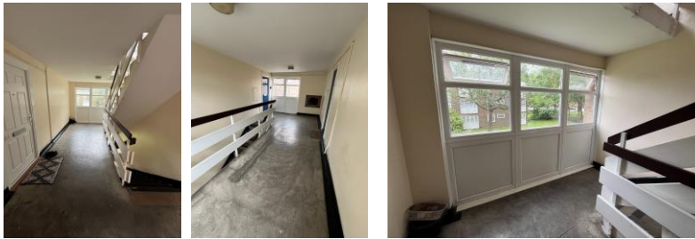
1st and 2 nd floor landing
