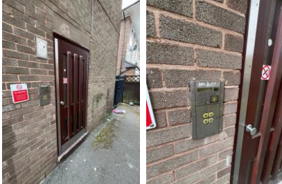
Entrance with door access control to the block
