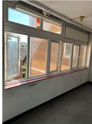
Manual window to flat lobby
