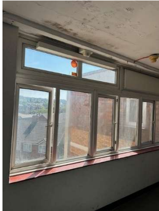
AOV window to flat lobby
