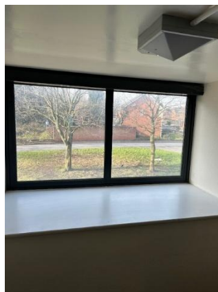
AOV window to staircase
