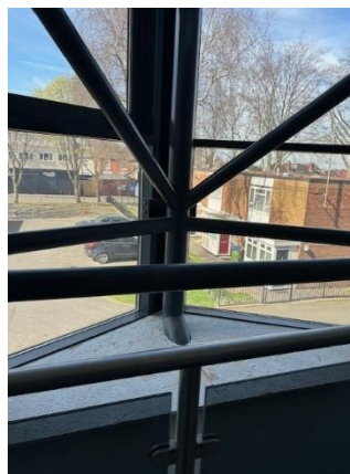
Fire stopped staircase base
