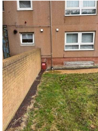
Dry riser inlet
