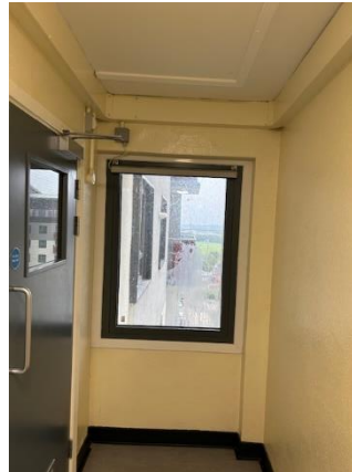
AOV window to corridor
