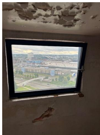
Manual opening window on staircase
