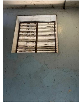
Vent to top of staircase (14 th floor)
