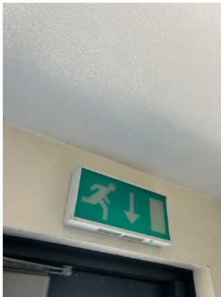
Bulkhead directional signage
