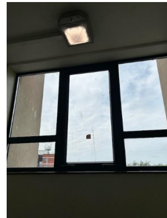
Manual opening windows to staircase
