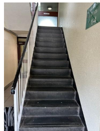
Front protected staircase
