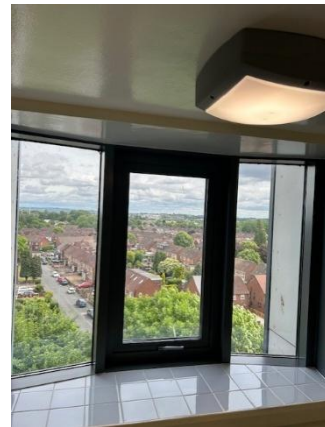
Manual windows to staircase
