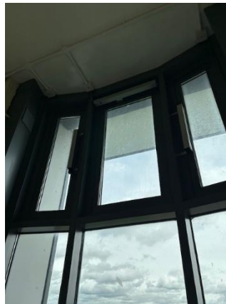
AOV windows (head of stairs)
