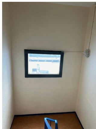
AOV window (16 th floor)
