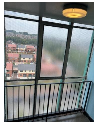
Fixed windows to staircase
