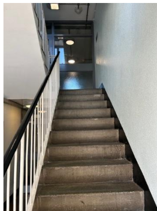
Front protected staircase
