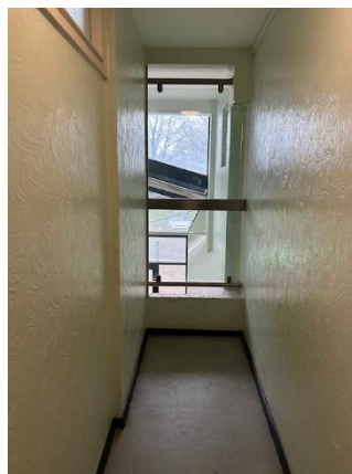
Open panel to staircase (1 st floor)
