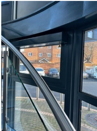
AOV window to basement
