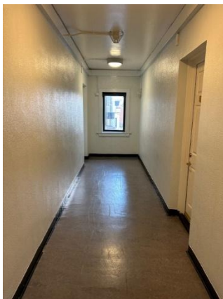
Dead-end with 19.5m travel distance (1 st floor)
