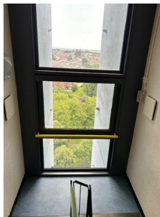
AOV window – floor 16
