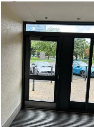
Ground floor exit
