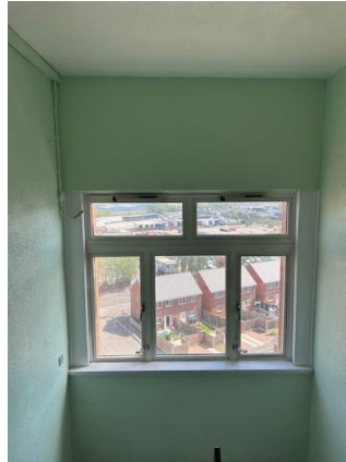
AOV window 7 th floor
