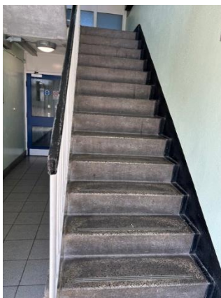
Front protected staircase
