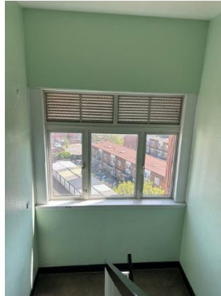
Manual window and fixed vent to staircase
