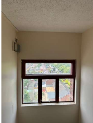
AOV window to staircase
