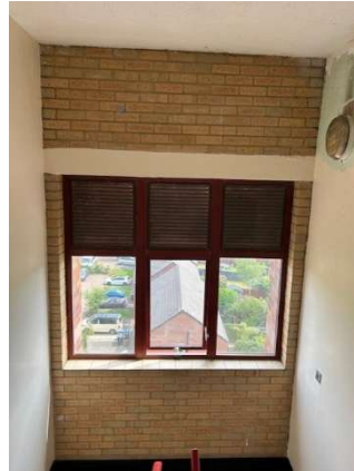
Manual window to staircase
