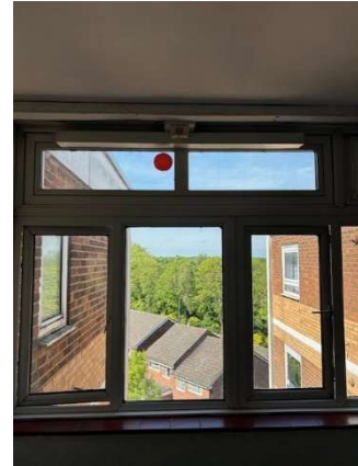
Ventilation grill (head of staircase) AOV window
