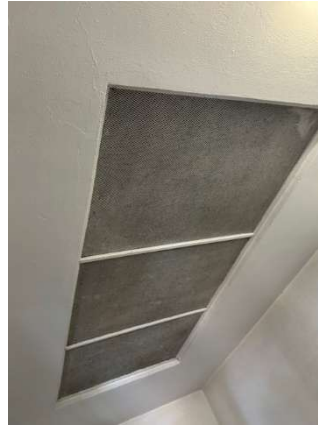
Ventilation grill (head of staircase) AOV window
