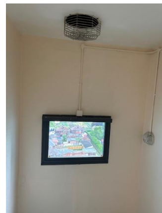
AOV window – 16 th floor
