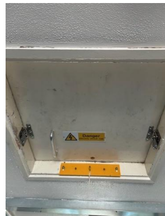
Hatch to lift motor room
