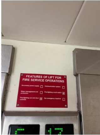
Lift information sign
