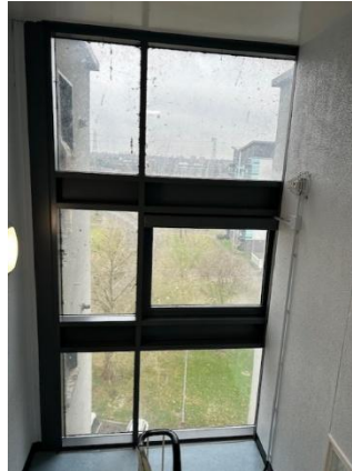
AOV window to staircase
