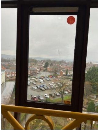
AOV window to staircase
