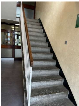
Front protected staircase
