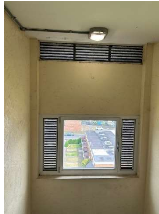
Manual window to staircase
