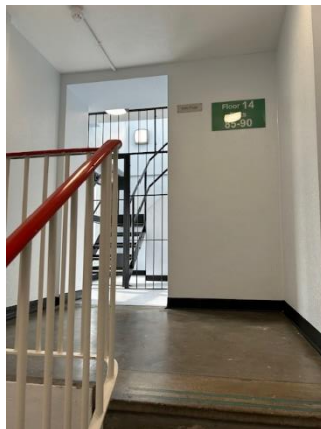
14 th floor staircase
