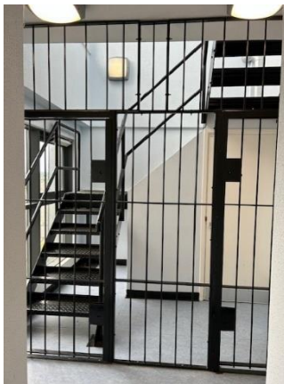
Security gate to enclosed roofspace
