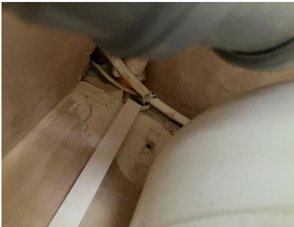
Figure 25: Flat service penetration
