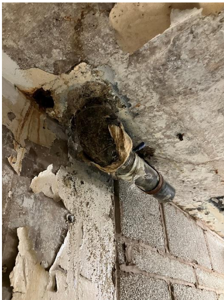
Figure 22: Pipework through floor slab
