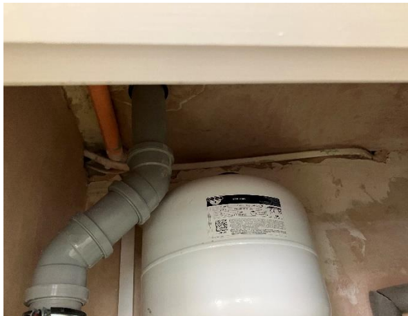
Figure 24: Flat service penetration
