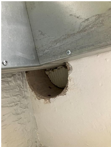
Figure 26: Floor slab of refuse room chute
