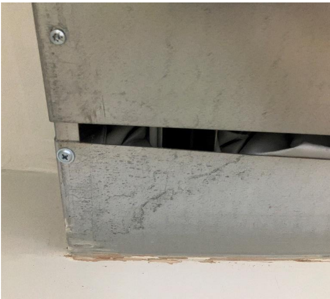
Figure 23: Exposed trunking
