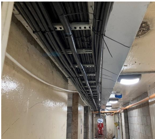
Figure 20: Cable installation LG
