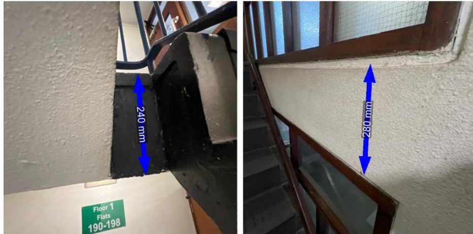
Figure 14 and 15: Slab edges including screed and finishes
