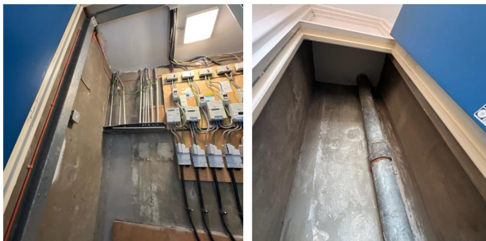
Figure 16 and 17: RC internal elements and communal space
