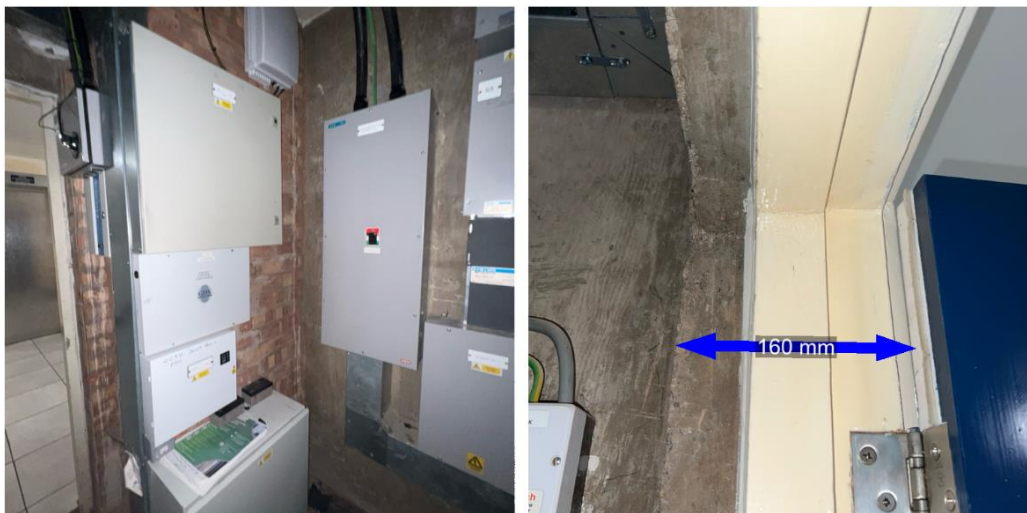
Figure 15 and 16: RC walls
