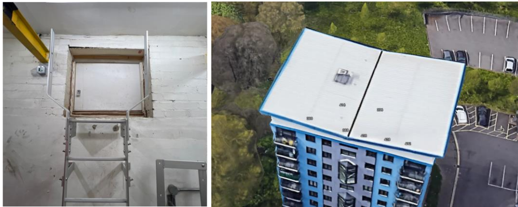
Figure 11 and 12: Access latch closed and Roof Level from satellite
