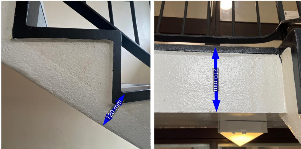
Figure 13 and 14: RC Staircase stringer and slab
