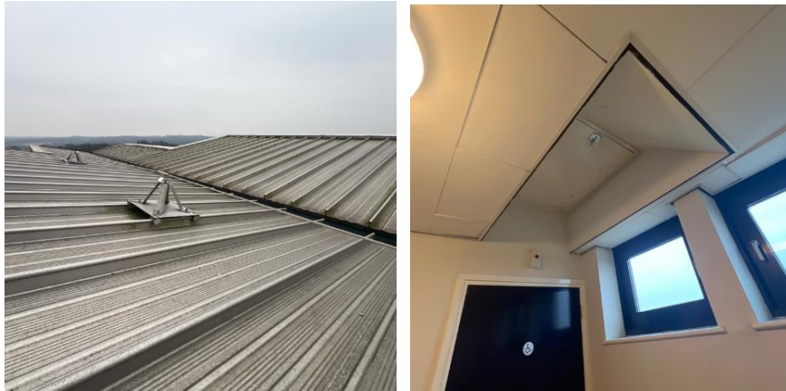
Figure 11 and 12: Roof Level
