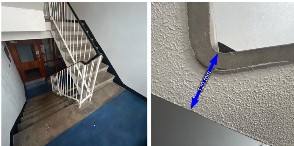
Figure 15 and 16: Stair stringer and staircase
