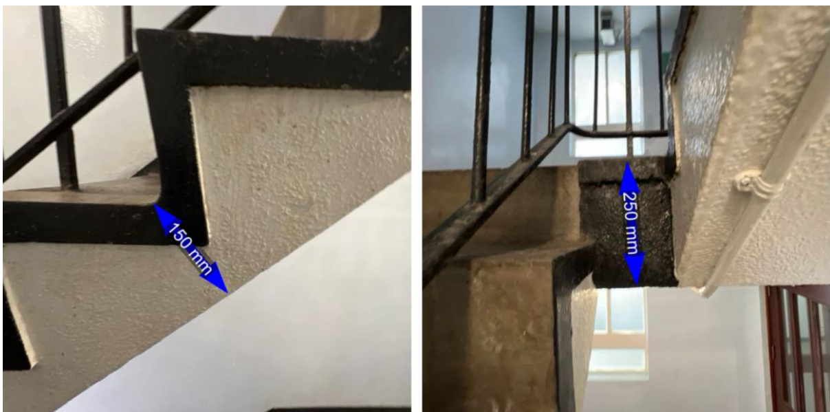
Figure 15 and 16: Staircase Stringer and shear wall
