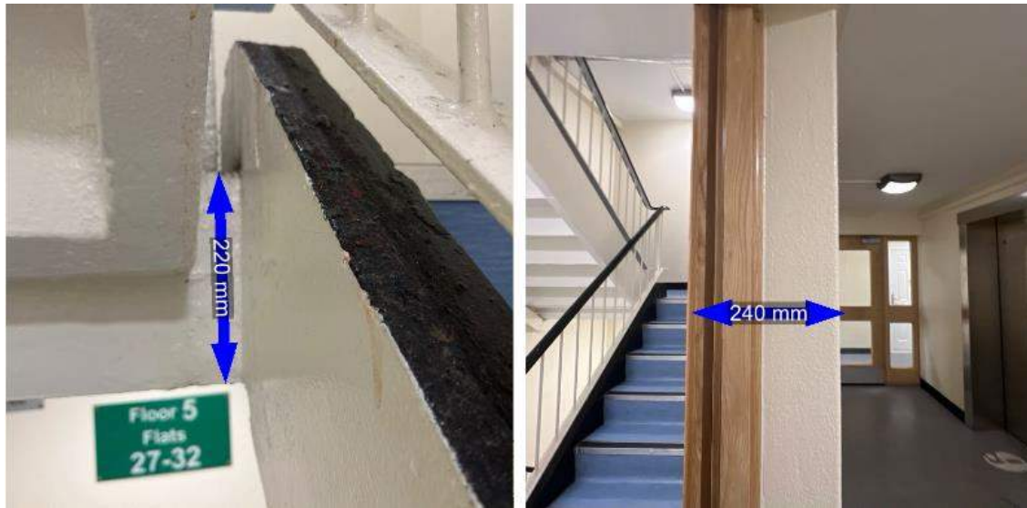
Figure 13 and 14: RC Structure
