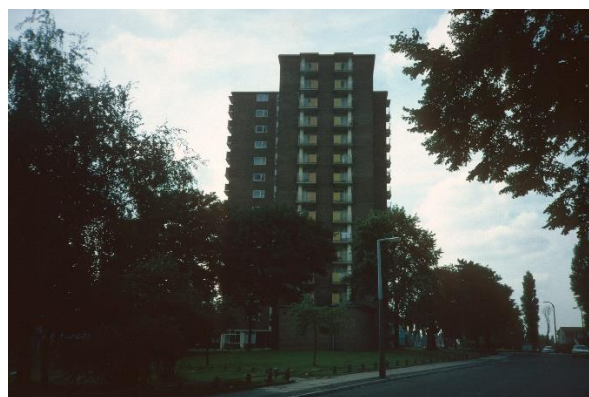
Figure 5. View of the Thompson Gardens prior to re-cladding
