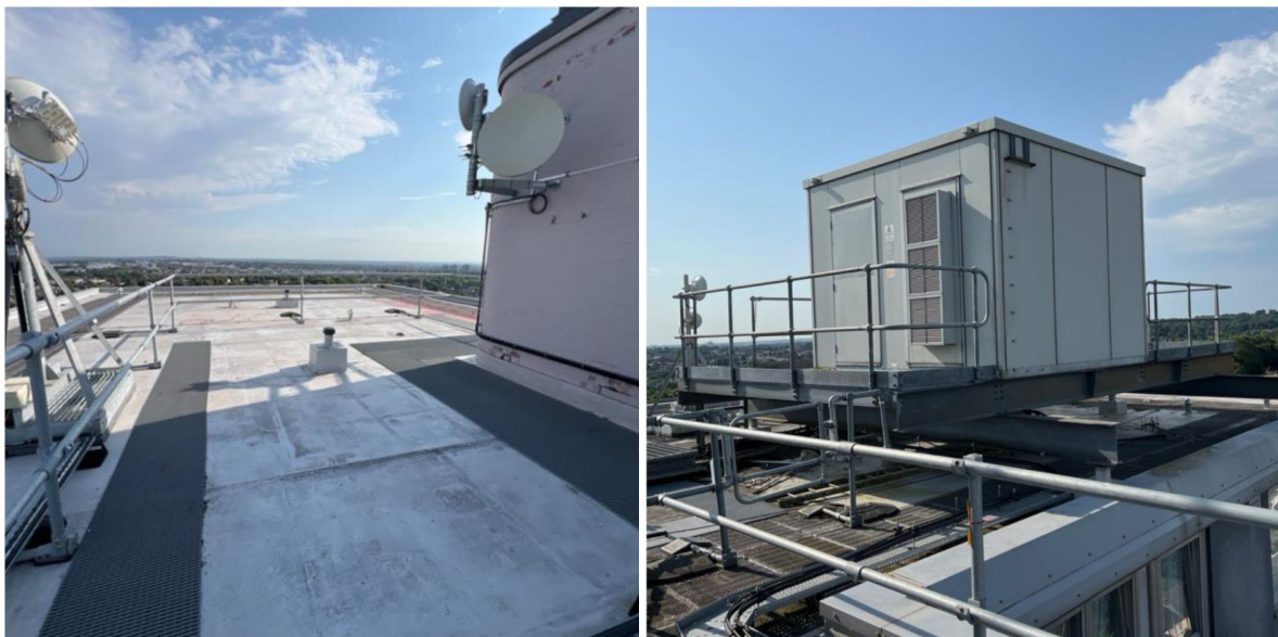
Figure 11 and 12: Roof Level
