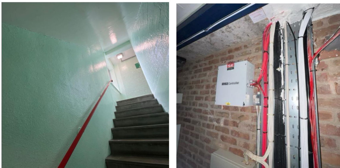
Figure 15 and 16: Staircase shear wall and masonry infill panels
