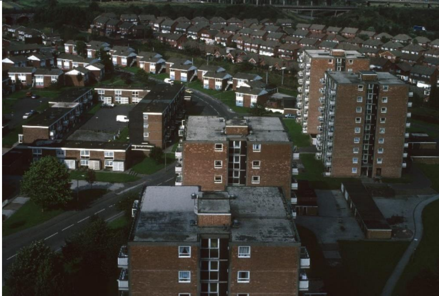
Figure 5. Charlemont Farm estate before the buildings underwent the refurbishment in 2015. Stanton House is third building on the right
