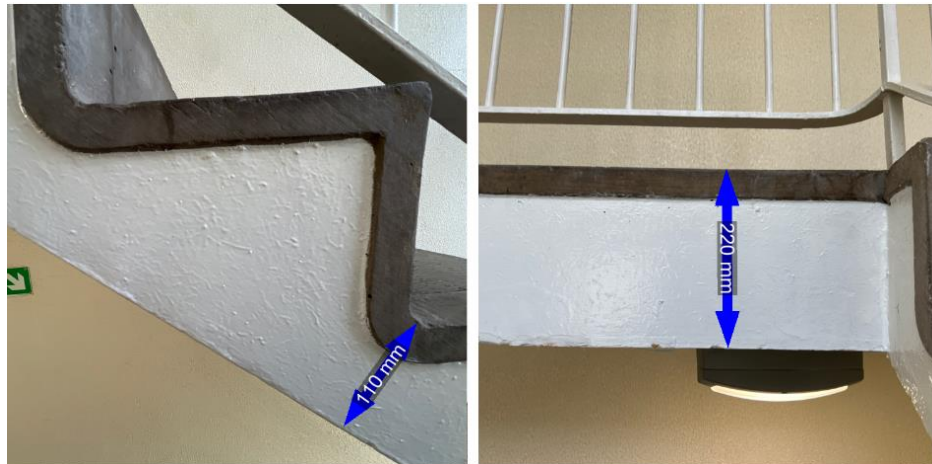
Figure 13 and 14: RC Staircase stringer and slab
