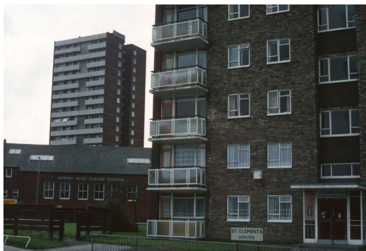
Figure 5. Building in background Before Cladding Refurbishment
