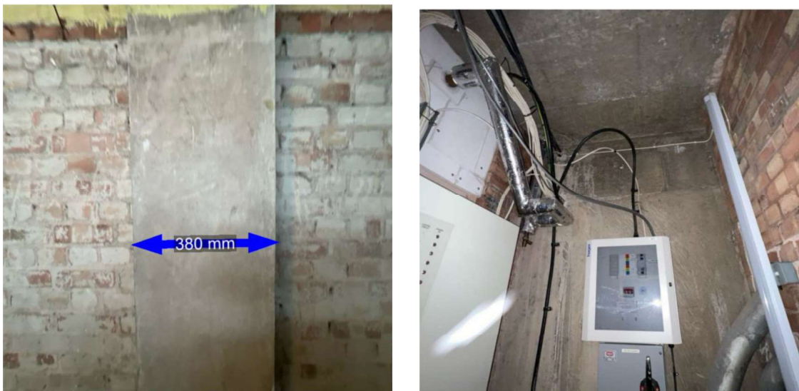
Figure 15 and 16: Internal RC Columns noted and vertical RC Structure
