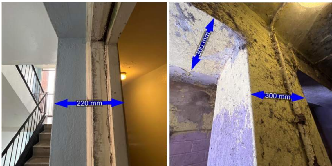
Figure 13 and 14: RC Structure
