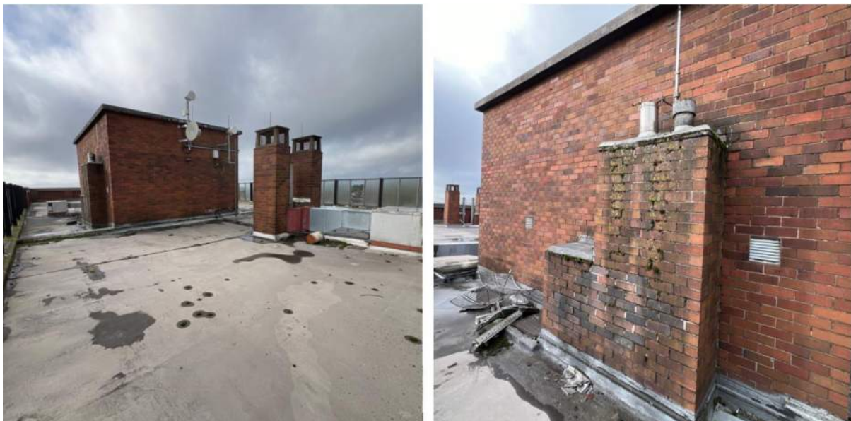
Figure 11 and 12: Roof Level
