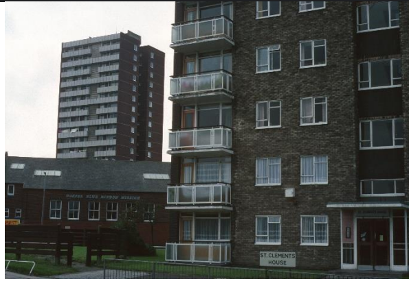
Figure 5. View of St Clements House before the building underwent the refurbishment in 2007
