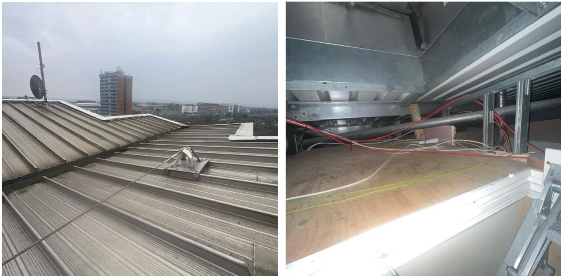
Figure 11 and 12: Roof Level
