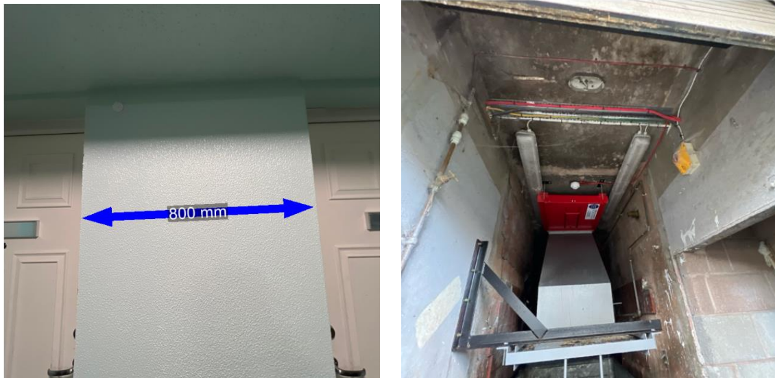
Figure 15 and 16: RC Column at typical level and slab viewed at GF
