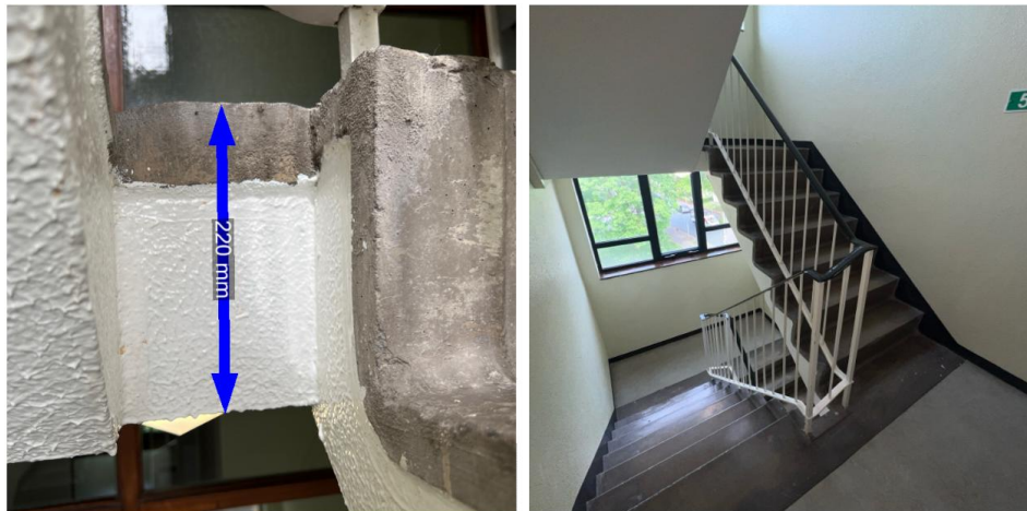
Figure 14 and 15: Slab edge and stair stringer
