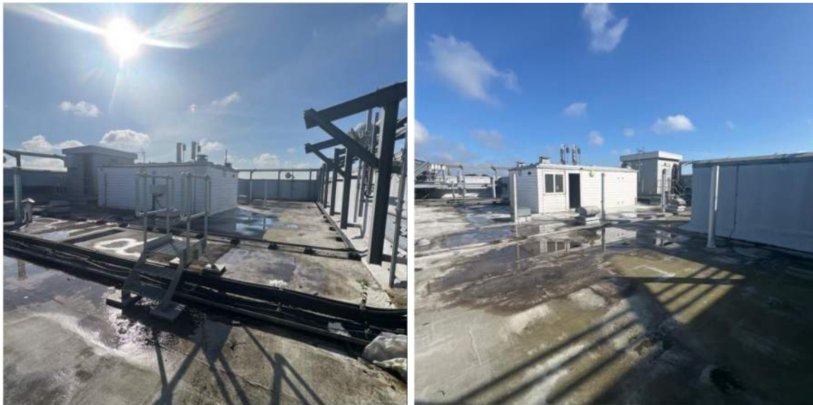
Figure 11 and 12: Roof Level
