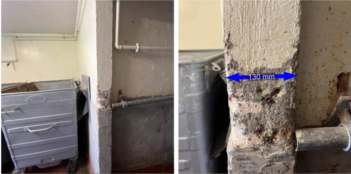
Figure 13 and 14: RC Structure
