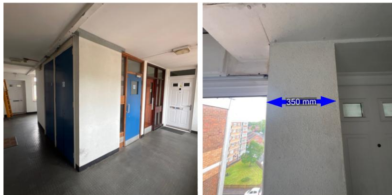
Figure 16 and 17: RC internal elements and communal space
