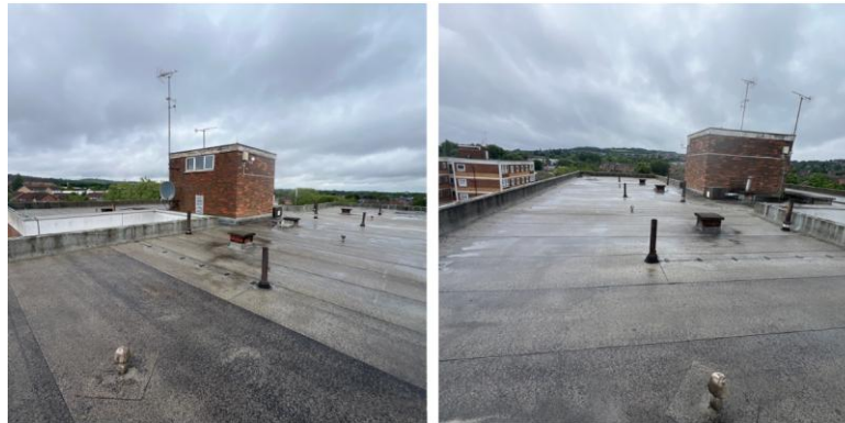
Figure 11 and 12: Roof Level
